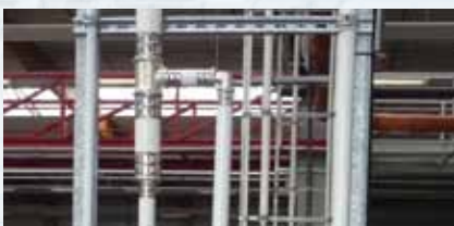
Compressed air installations
